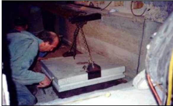
Figure 1. Installation of ceramic tiles in a furnace hearth at Indalco.
